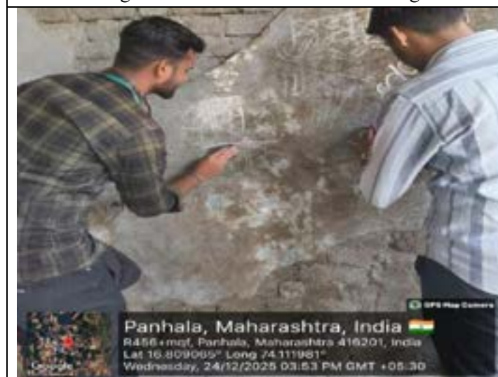
Cleaning of Temple Walls within Fort Premises
