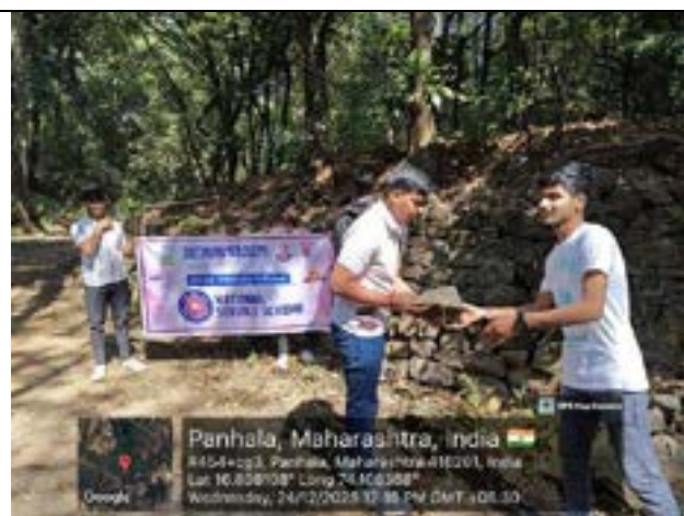
Conservation Work by Placing Displaced Stones Properly
